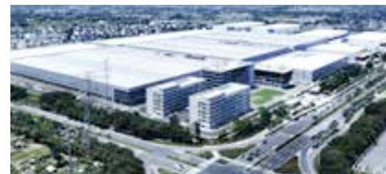
PV Module Manufacturing Base
