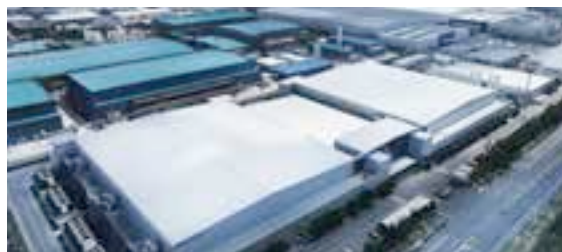
PV Wafer Manufacturing Base
