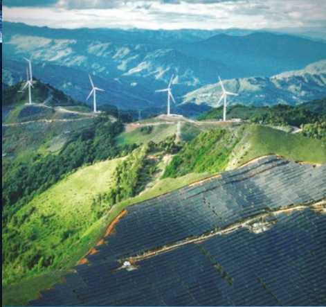
Utility-Scale PV Power Plants
