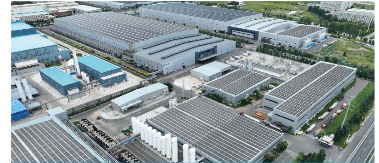
PV Wafer Manufacturing Base
