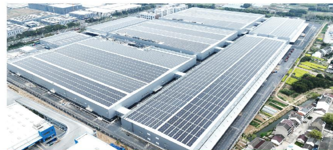
PV Module Manufacturing Base
