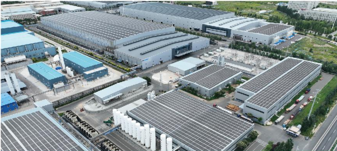
PV Wafer Manufacturing Base
